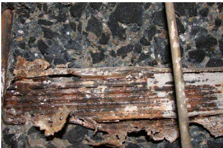
**Figure 12:** Corroding prestressing steels after opening of the duct
