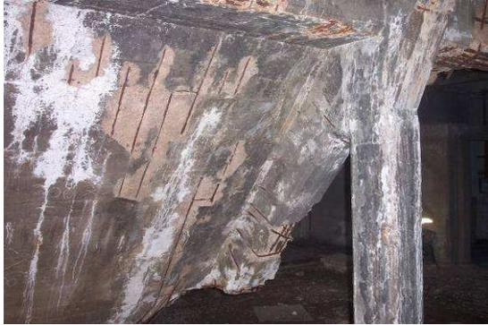
**Figure 3.** Corrosion of the reinforcement of an old concrete structure caused by insufficient concrete cover
