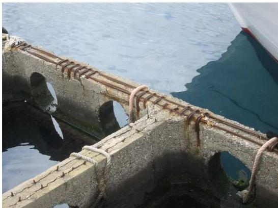
**Figure 1.** Example for chloride induced reinforcement corrosion in concrete exposed to seawater
