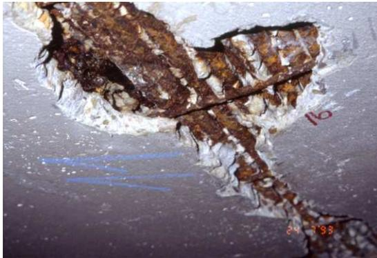
**Figure 4.** Corrosion of the reinforcement caused by local bad compaction of the concrete
