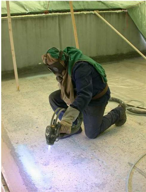
**Figure 8.** Sacrificial cathodic protection of steel in concrete by thermal zinc spraying
