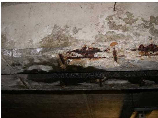
**Figure 2.** Example for chloride induced corrosion of the reinforcement exposed to deicing salts within a leaking joint of a parking garage
