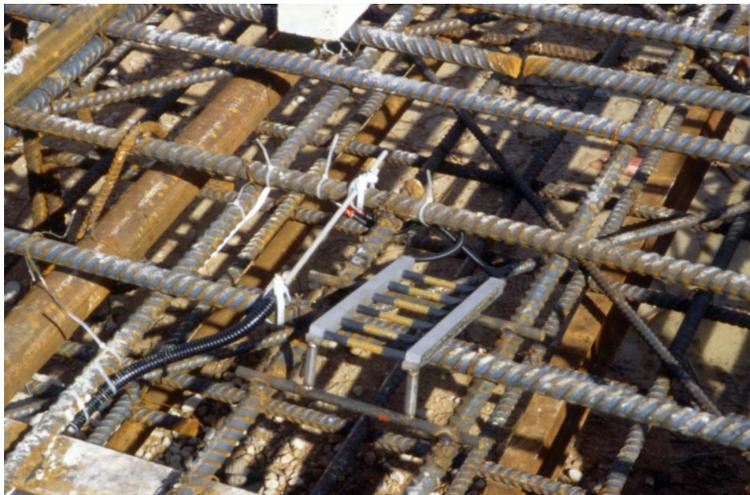
**Figure 13.** Sensors installed in a concrete structure to monitor the corrosion risk for the reinforcement
