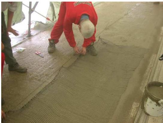
**Figure 9.** Cathodic protection by an impressed current using a carbon mesh anode in a special mortar
