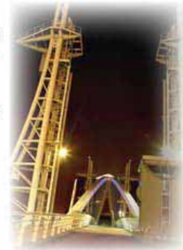
The Lowry Road bridge, Salford Quays
