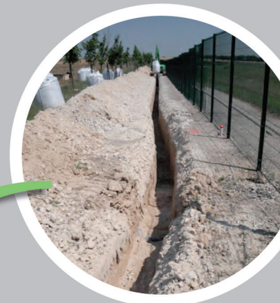
Anodes installation on coke breeze bed
