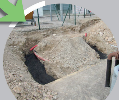
Anodes installation on coke breeze bed
