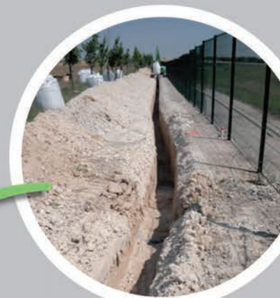
Anodes installation on coke breeze bed
