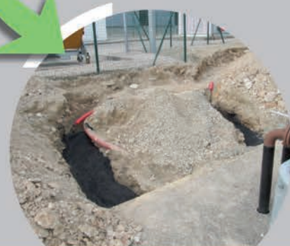
Anodes installation on coke breeze bed
