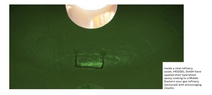
Oil and gas facilities, especially gas sweetening plants, are prone to extreme corrosion, particularly within amine sweetening units, but HEGGEL have produced a hybridized epoxy coating that has provided a sustainable protection solution at a Middle Eastern sour gas refinery.
