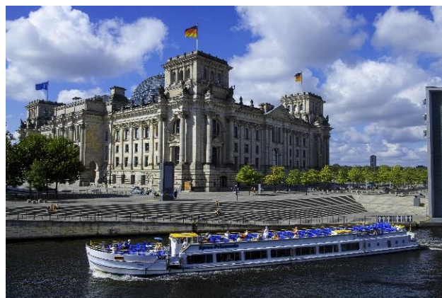
Exterior of Reichstag building (Copyright: visitBerlin, Foto: Artfully Media, Sven Christian Schramm)
