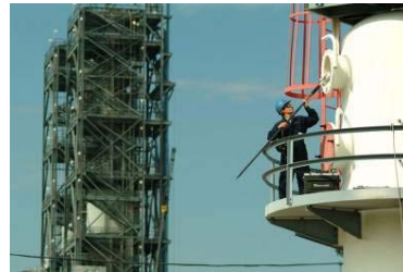
Refinery Distillation Tower Inspection
