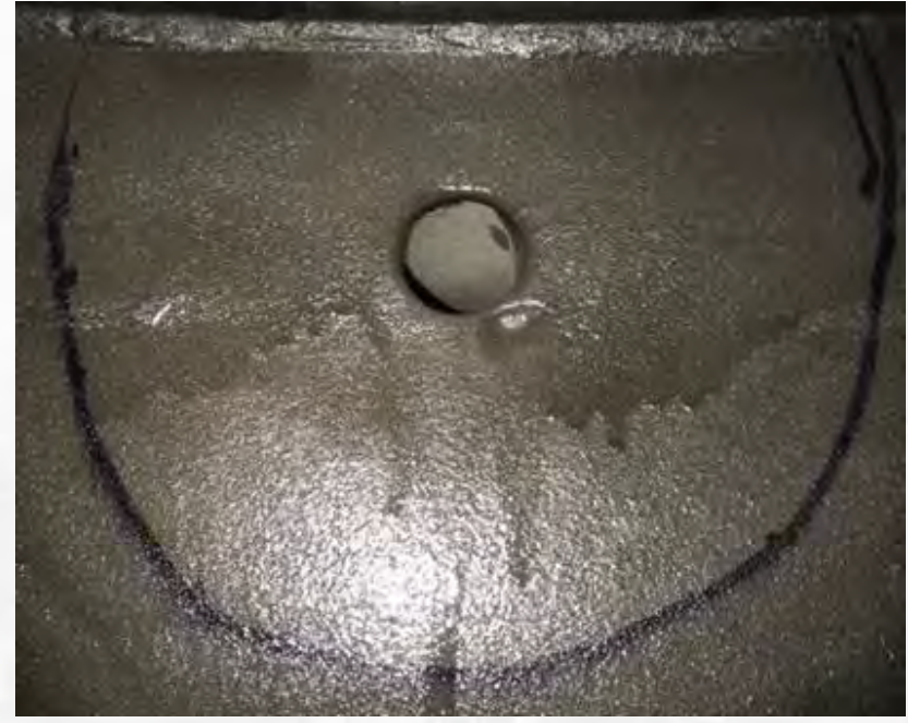
Nozzle after HVTS application
