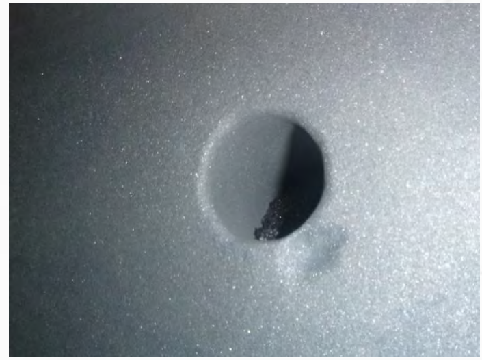
Nozzle after surface preparation
