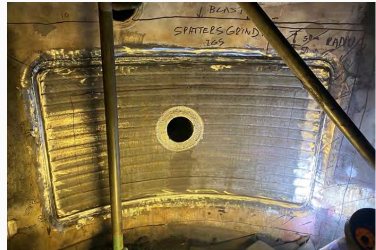
Plate after installation
