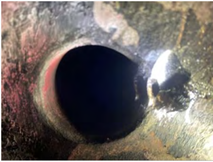
Nozzle after grinding
