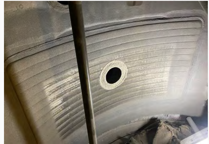
Plate after surface preparation
