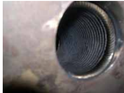
Automatic Overlay inside Vessel bores and nozzles
