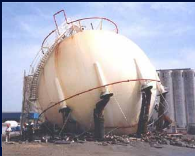
In-service Integrity Inspection
