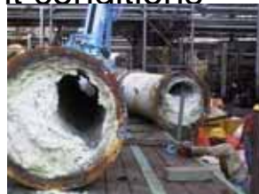
Accumulation of condensation debris in duct
