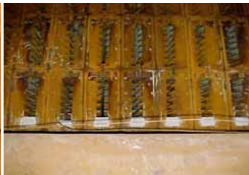
Air side repair
