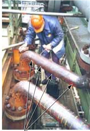
PEC monitor points (12 per pipe)
